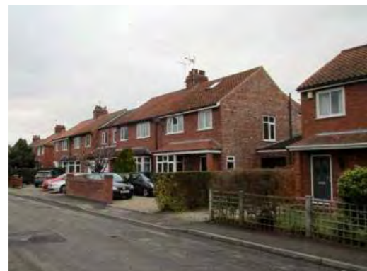
Photo 25: Housing on Moor Lane
