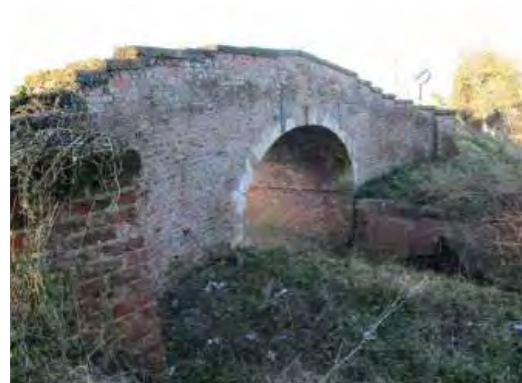
Photo 9: Strensall New Bridge
