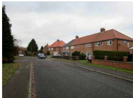
Photo 29: Housing on Northfields
