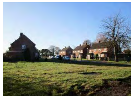
Photo 18: Housing along St Wilfred's Road
