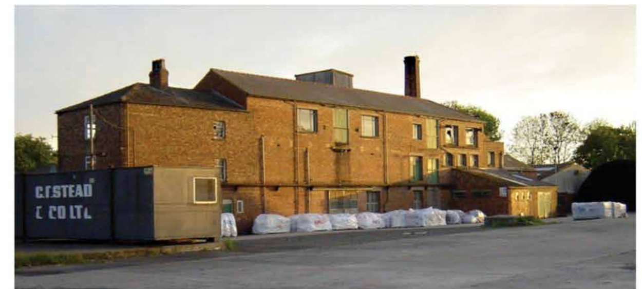
The Tannery, Strensall, now demolished
