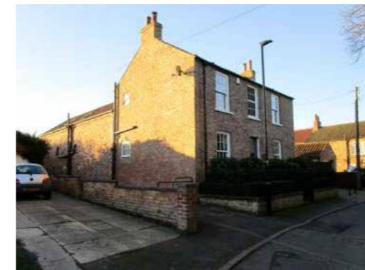
Photo 34: Example of detached house with rear wing
