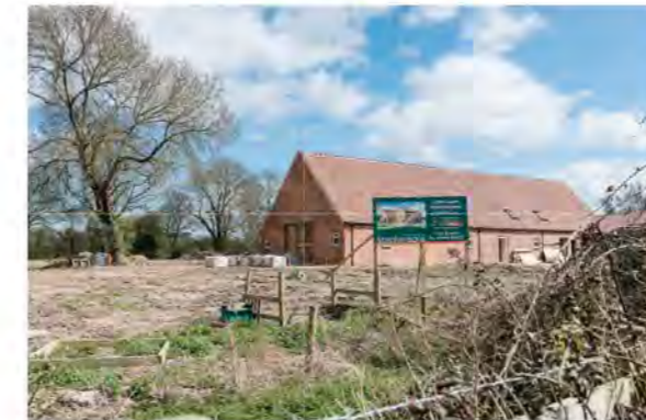
Towthorpe: conversion of agricultural buildings
