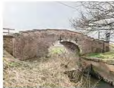
Strensall New Bridge – Haxby Moor Road
