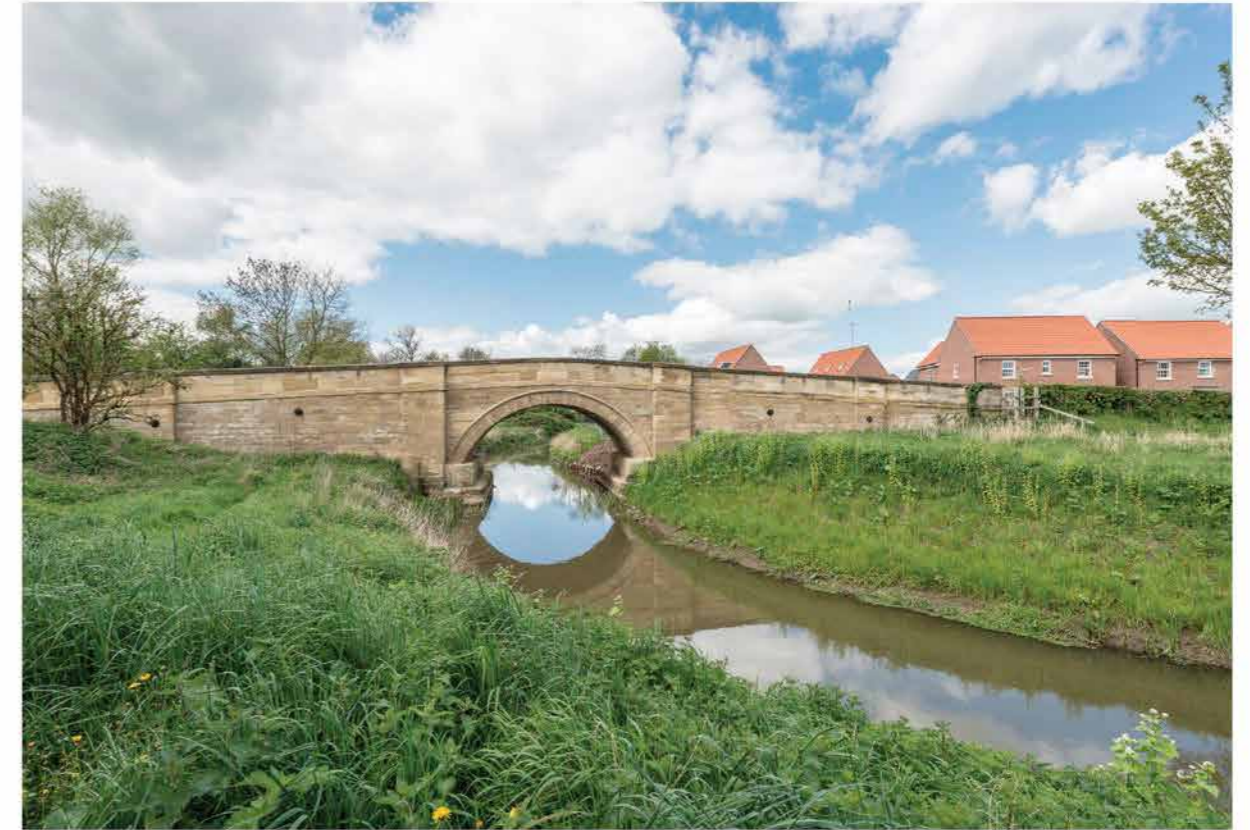
c2. West towards John Carr's bridge
