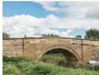
Strensall Bridge – Sheriff Hutton Road
