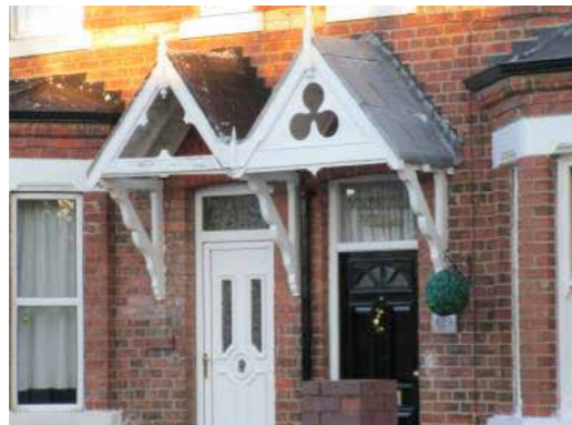
Photo 45: View of decorative detailing
